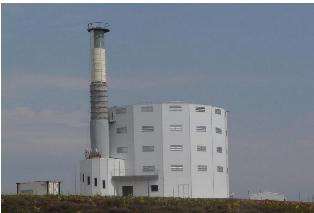
SALT building construction as at 15 October 2001 (photograph SALT)
